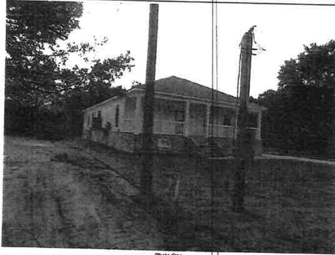
Photo One Caption 09/09/2019 NORTHWEST CORNER
