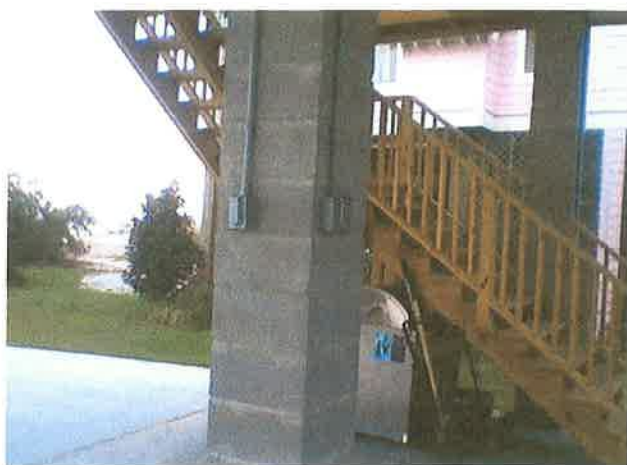
ELECTRICAL OUTLETS 16.47FT. 9-5-14
