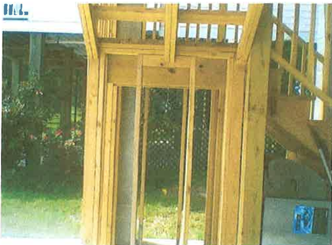
FRAMED AREA UNDER STAIRWAY 9-5-14
