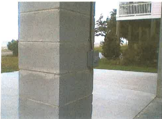
SWITCH FOR CARGO LIFT 15.17FT. 9-5-14
